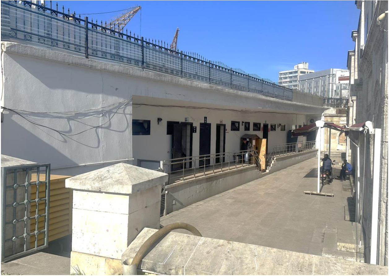
Figure 26 Site Photos, Public Restroom Facility
